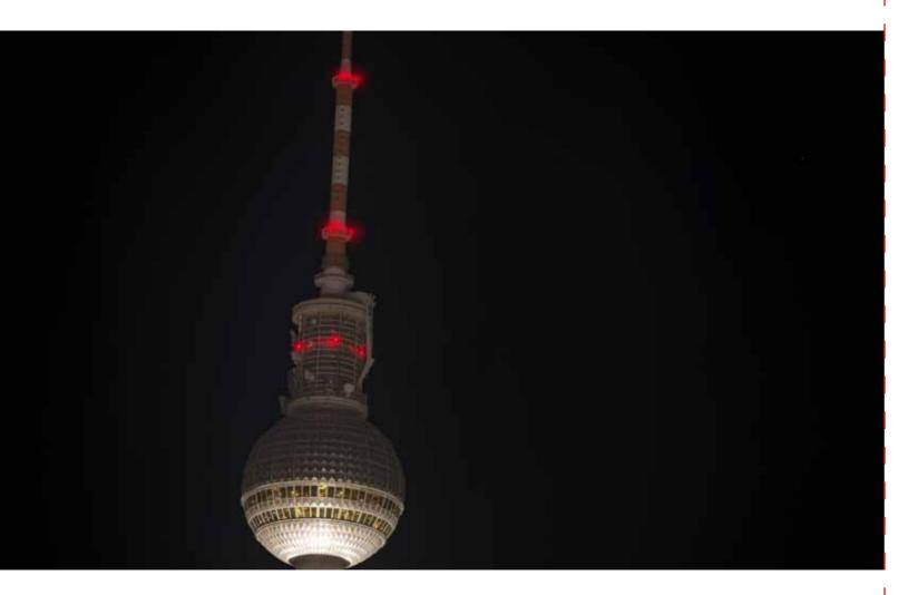
Obstruction lighting is crucial to tall structures, buildings, and airports around the world. A legal requirement, it marks the presence of all tall structures that may be a hazard to air navigation at night. The lighting system must be designed to meet International Civil Aviation Organization (ICAO) standards for product specification and placement to meet the highest levels of safety and visibility.
